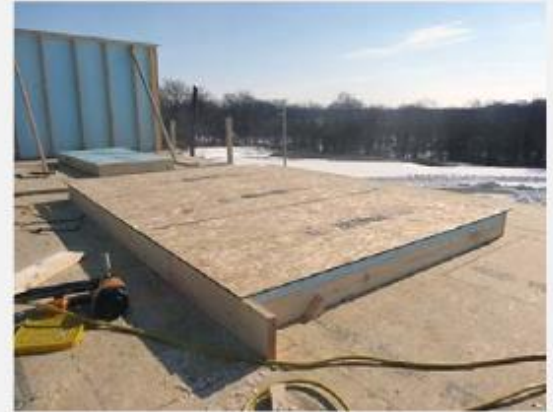
Sheathing over foam wall assembly
