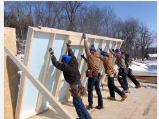
Typical wall section installation
